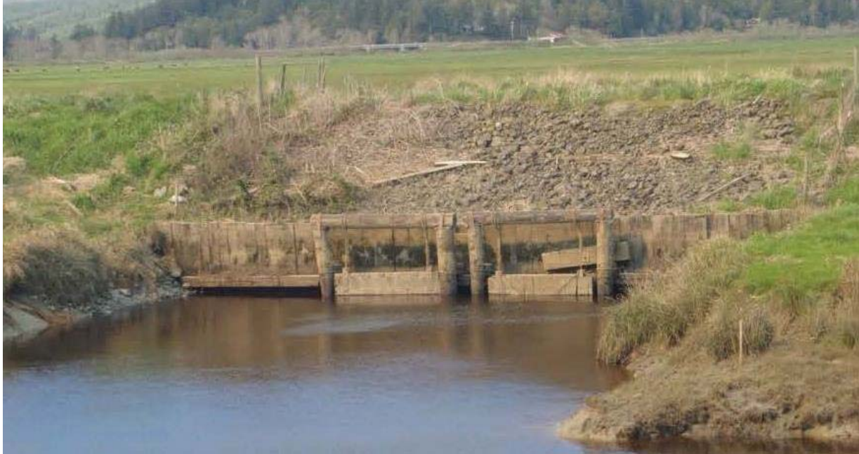
Figure 6. Existing Project tide gate infrastructure.
